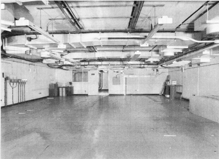
Upper floor - One of the many empty equipment rooms - Photo by Nick Catford
